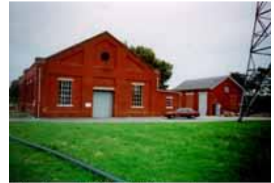
Fig. 2 Existing buildings at Manchester-Davyhulme WWTP from the times of Arden and Lockett
